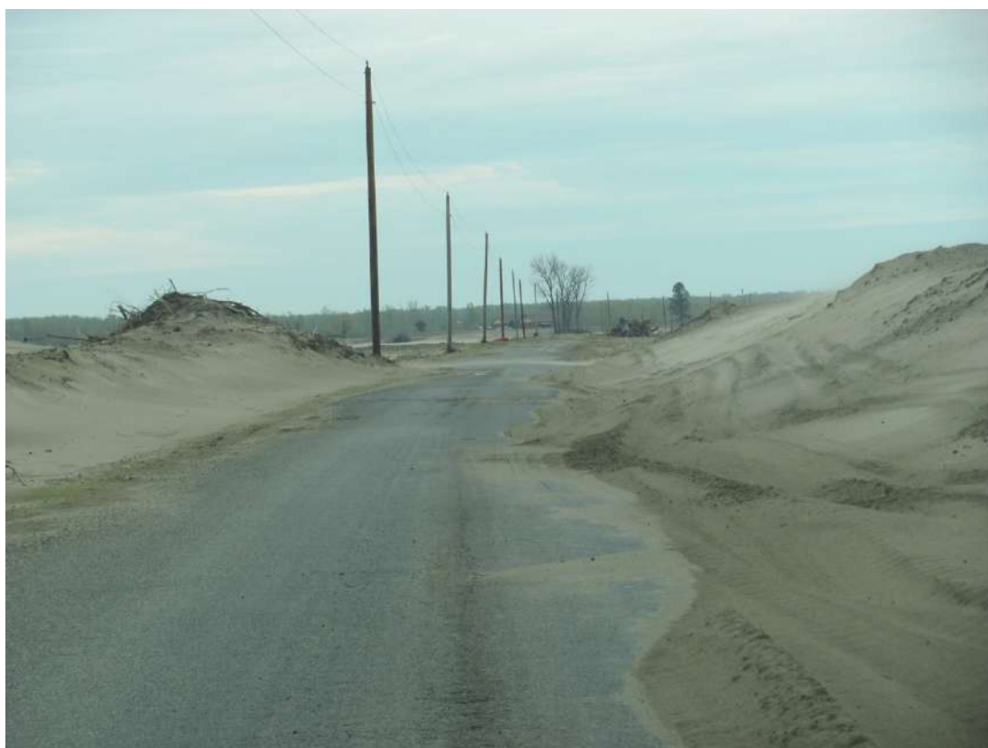
Figure PD14. Sand deposited by Mississippi River floodwaters after a Len Small levee breach in 2011. The sand had to be removed by a grader and a snowplow. Reprinted with copyright permission of the Editor of the Open Journal of Soil Science.
