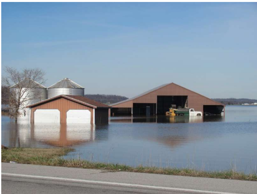
Figure PD7. Flooding along Illinois Highway 3 near the Len Small levee breach. The entire farmstead was covered by Mississippi River floodwaters in 2011. Reprinted with copyright permission of the Editor of the Open Journal of Soil Science.
