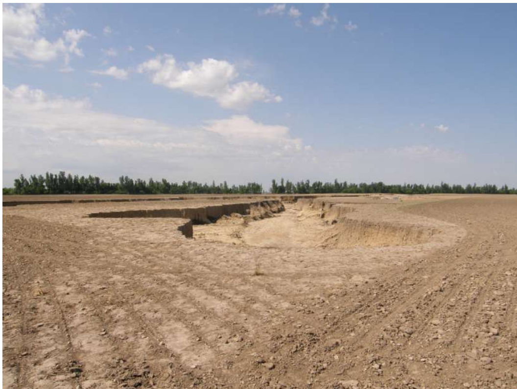
Figure PD13. Deep gully in a cultivated field on O'Bryan Ridge created by water rushing through the made-made Birds Point levee breach. Reprinted with copyright permission of the Editor of the Open Journal of Soil Science.
