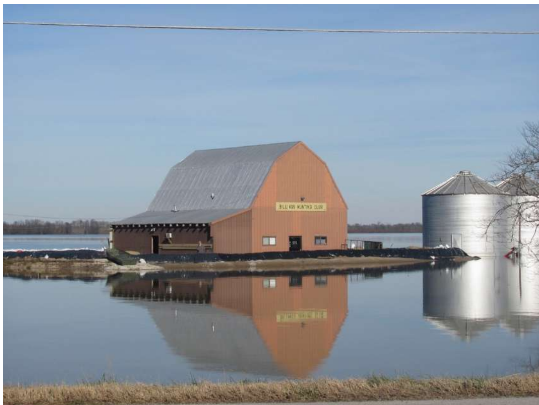
Figure PD5. A picture of a private levee protected barn. The man behind the levee is on his cell phone. Reprinted with copyright permission of the Editor of the Open Journal of Soil Science.
