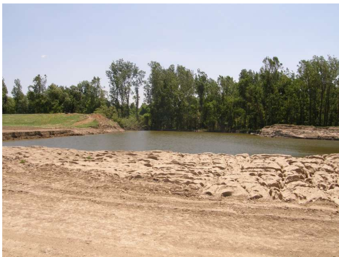
Figure PD8. The first, of three Birds Point levee breaches, was triggered by the use of TNT by the US Army Corps of Engineers. The crater lake is between the levee and the adjacent farmland. Reprinted with copyright permission of the Editor of the Open Journal of Soil Science.
