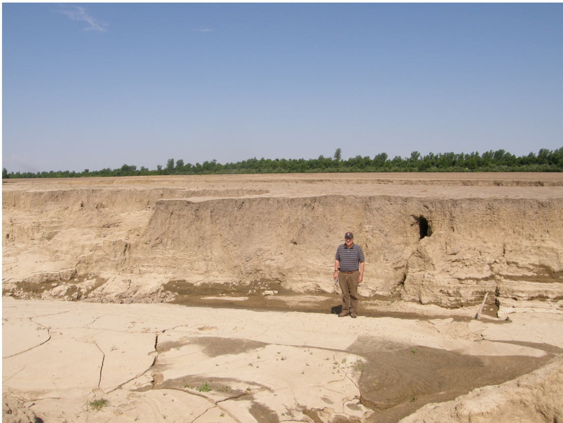
Figure 4. The first of three Birds Point levee breaches was triggered using TNT by the U.S. Army Corps of Engineers. The crater lake is between the levee and the adjacent farmland. Photo credit: Kenneth Olson. Reprinted with copyright permission of the Editor of the Open Journal of Soil Science.
