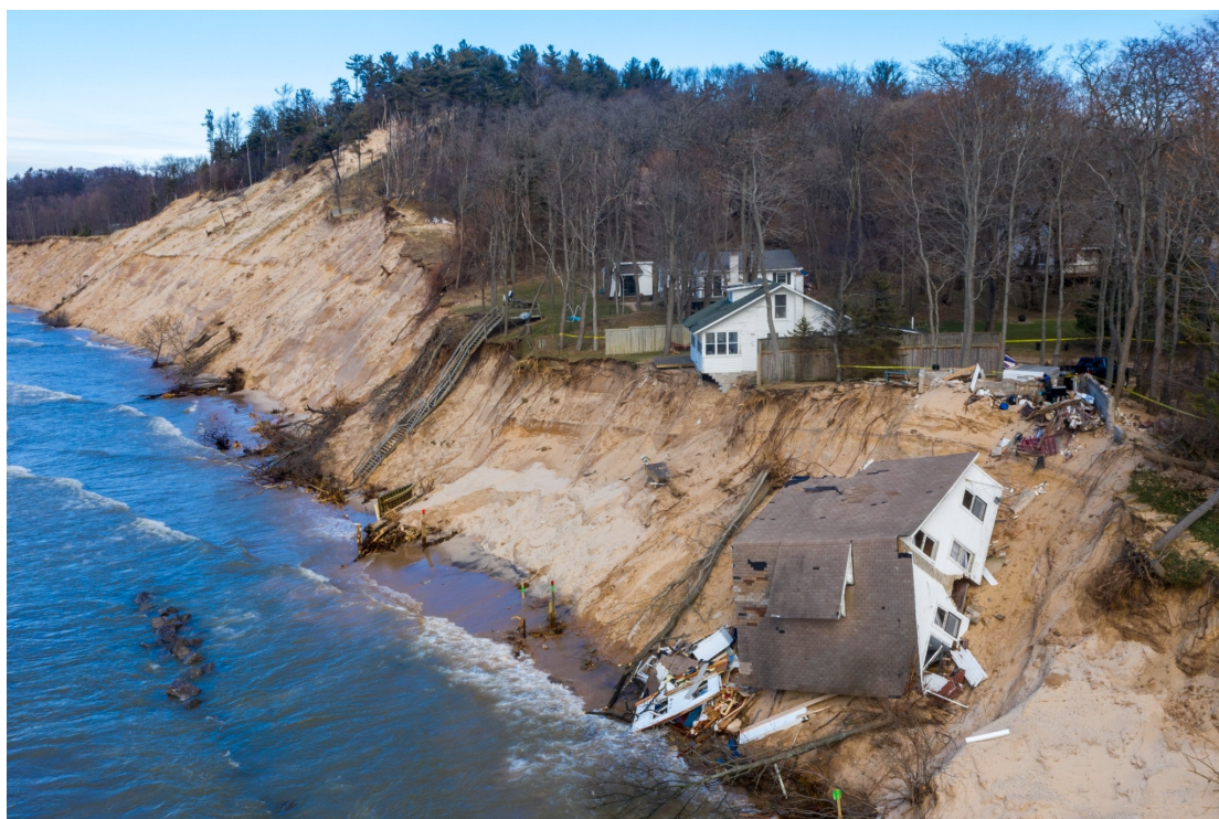
Figure 5. Shoreline erosion undercutting the shore and damaging a beach house on Lake Michigan. Photo credit: 2020 MLive Media Group. Reprinted with copyright permission from the Managing Editor of the Open Journal of Soil Science.
