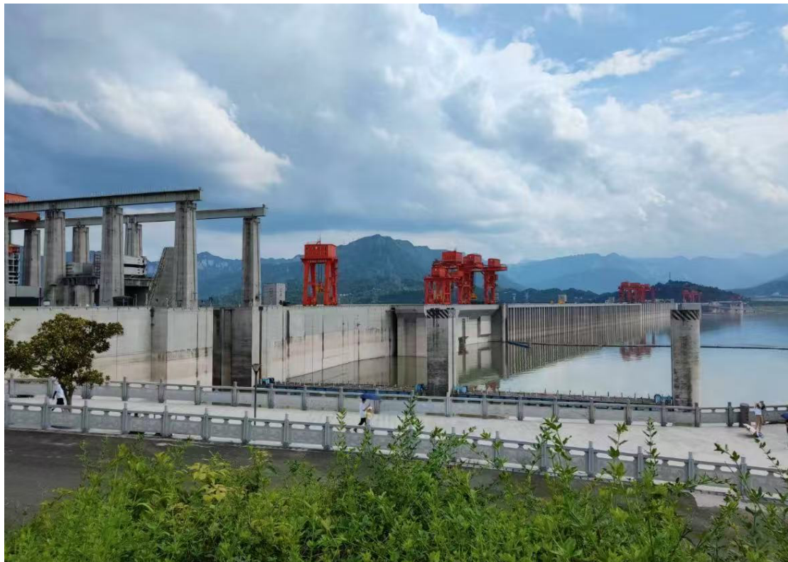
Figure 5. Three Gorges Dam on the Yangtze River. Photo credit: Wadslin Frenelus.
