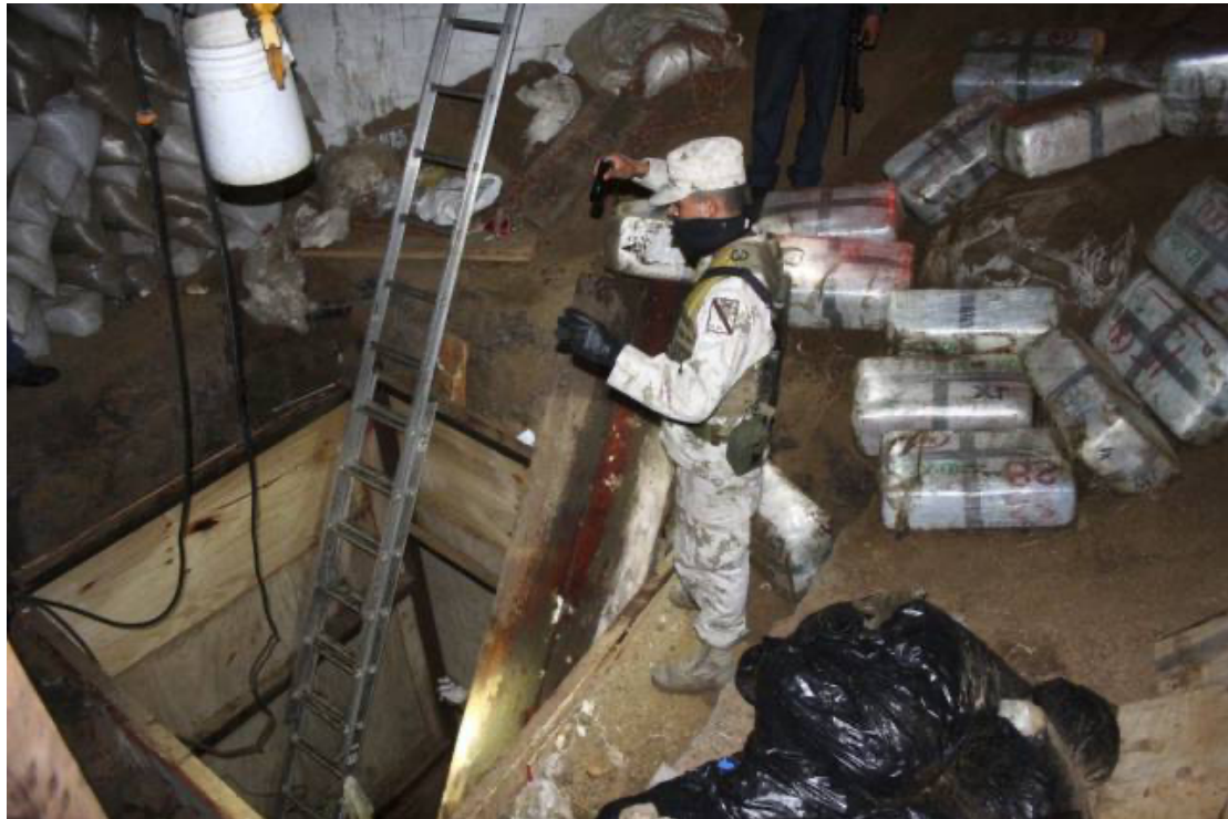
Figure 3. Soil tunnel shaft used to access the tunnel 10 m below the soil surface. The drug packages are lifted by a pulley system. Reprinted with copyright permission of the Managing Editor of Open Journal of Soil Science.
