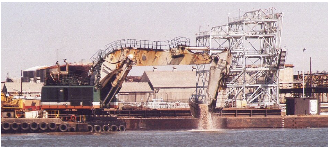
Figure 19. Deepening the Kill Van Kull channel to 17 m. USACE dredge brings up debris from bedrock broken by dynamite. Photo credit: Bob King.
