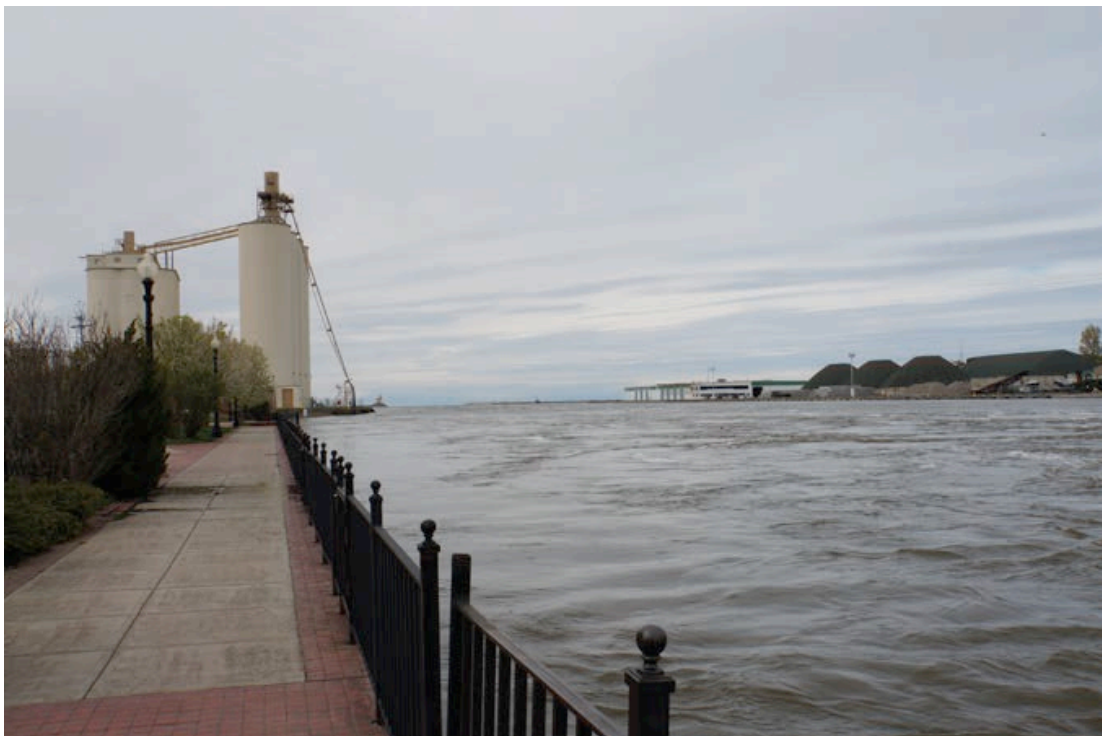
Figure 12. New York State funded construction of two modern grain elevators in the early 1900s. One was built at the port of Oswego on Lake Ontario enabling the transfer of agricultural fertilizers, grains, and other commodities; the other was the Gowanus Bay terminal in New York City (8).
