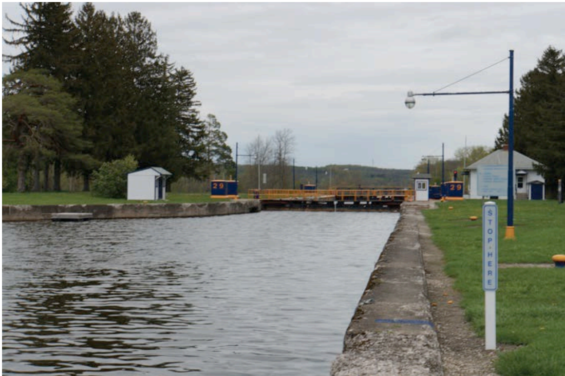
Figure 9. The gates are closed at Palmyra Lock 29 creating slack water in the foreground as canal boats approach the lock from the east (8).
